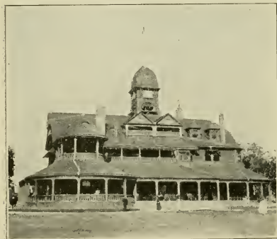
Casino, Belle Isle Park.
